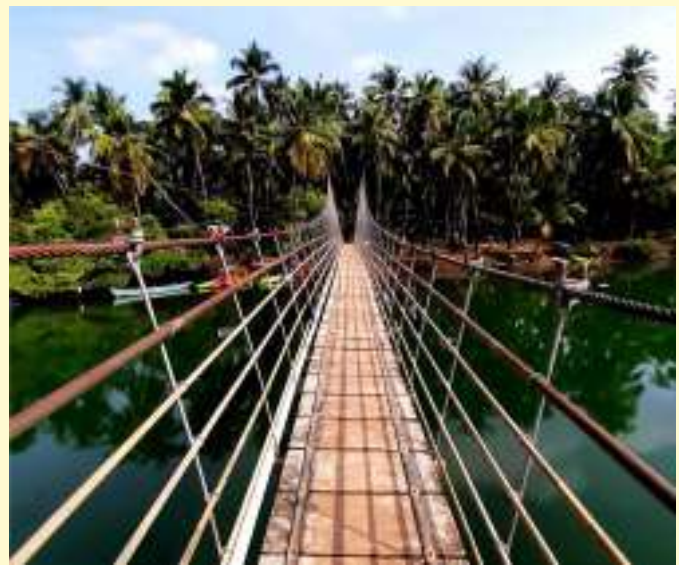
Kemmanna Hanging Bridge, Udupi
